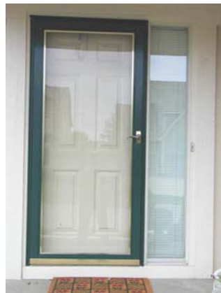
The snap on cover conceals the “retro-fit” security product from view (right)
