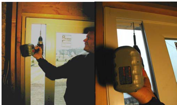
Screws are placed just above the door in the header, eliminating upward motion.
